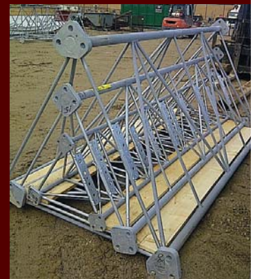
Tower ships nested to minimize freight
