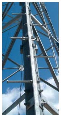
Welded Sections used on sections #13-21
